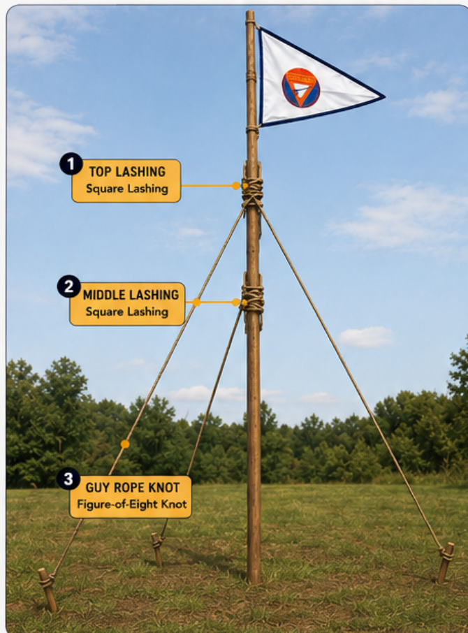
Figure-of-Eight Knot (Guy Ropes)
